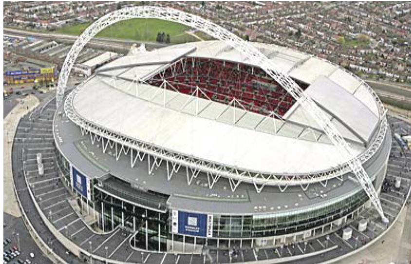
Exhibit 3 – The completed stadium
