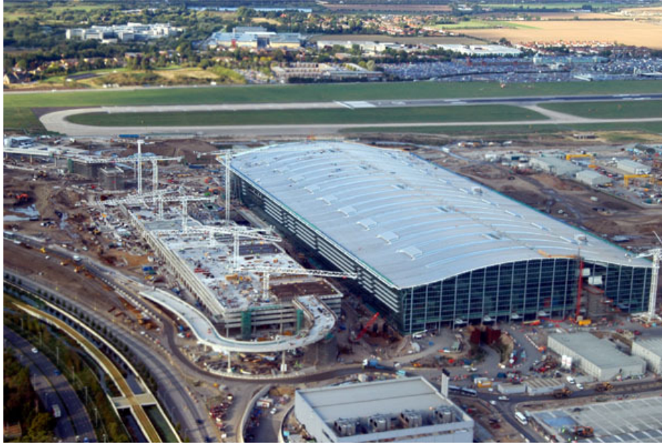
Exhibit 4 – T5 under construction, September 2005
