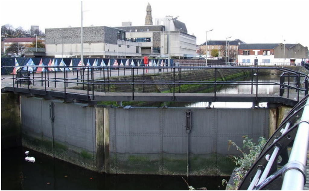
A set of mitre gates with a stone lined dry dock behind.
